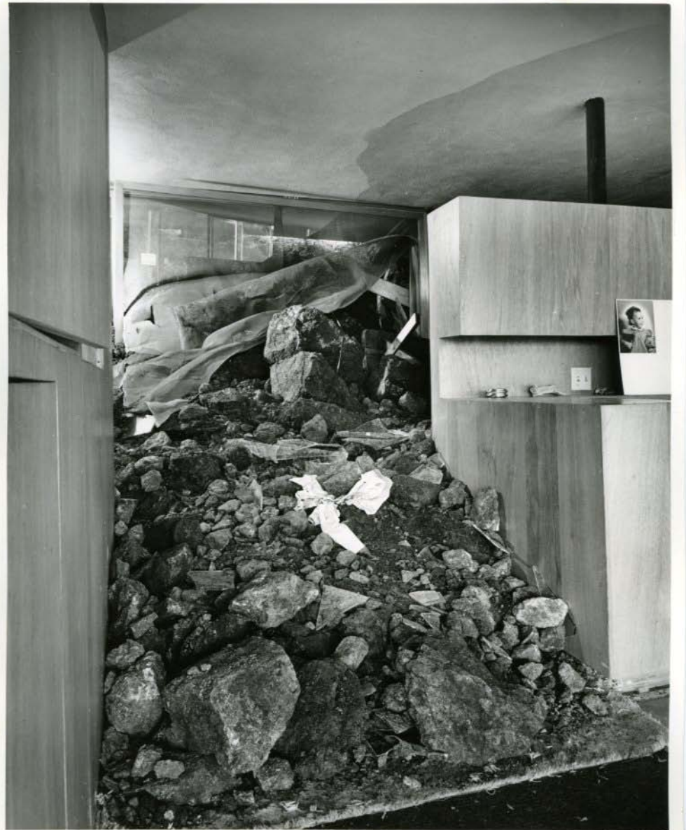
The living room of the Shulman residence invaded by a landslide, 1952.
