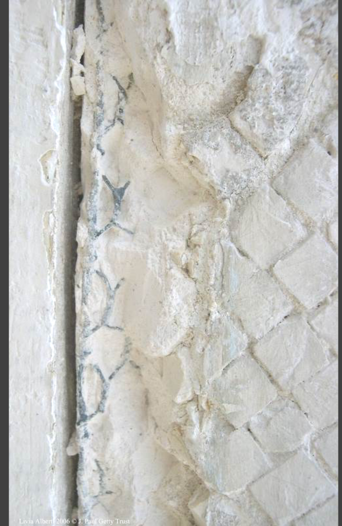
Steel wire grid
