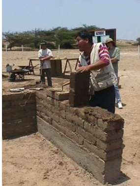
Figure 3.3.7 (left), 3.3.8 (center) and 3.3.9 (right) PAT instructor demonstrating adobe construction (left), students practicing rammed earth construction (center) and PAT instructor and mason working on a "quincha" model (right) PAT course, 1999 © J. Paul Getty Trust
