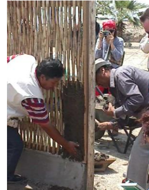
Figure 3.3.7 (left), 3.3.8 (center) and 3.3.9 (right) PAT instructor demonstrating adobe construction (left), students practicing rammed earth construction (center) and PAT instructor and mason working on a "quincha" model (right) PAT course, 1999 © J. Paul Getty Trust
