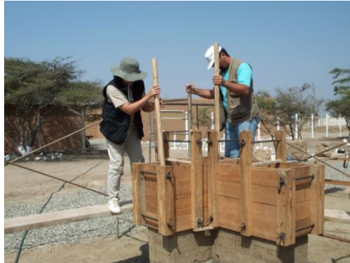
Figure 3.3.7 (left), 3.3.8 (center) and 3.3.9 (right) PAT instructor demonstrating adobe construction (left), students practicing rammed earth construction (center) and PAT instructor and mason working on a "quincha" model (right) PAT course, 1999 © J. Paul Getty Trust
