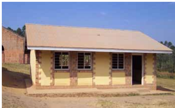
FIGURE 5 Prototype de construction contemporaine en adobe, Bushenyi, Ouganda, 2005. Photo : Olivier Moles. © CRATerre
