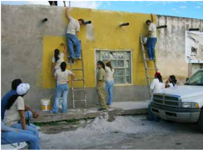
FIGURE 5 Architecture students applying the traditional lime paint, Ciudad Guerrero, Chihuahua, Mexico. Photo: Francisco Uviña, 2006
