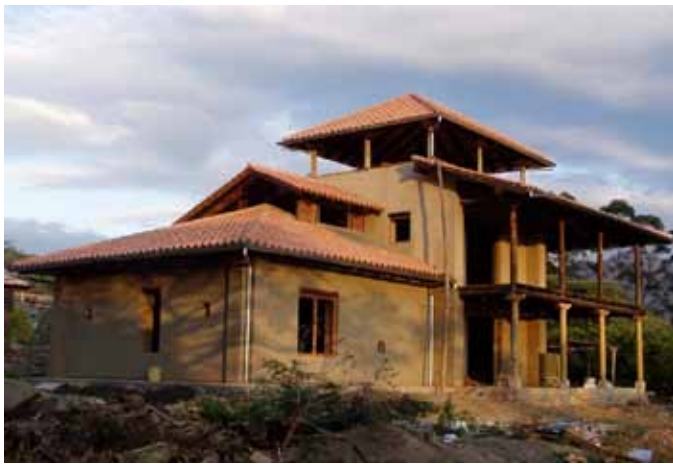
FIGURE 4 The Yunguilla House during construction. Photo: Lourdes Abad R., 2005
