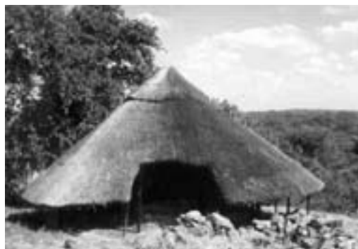
FIGURE 5 Roofing of the structure eliminates the threat of rain and direct sun but not the problem of humidity. Photo: Ashton Sinamai
