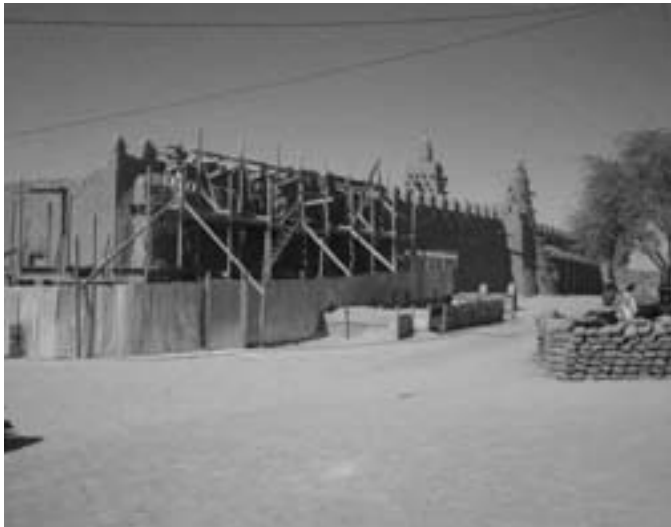
FIGURE 3 View of the Djingareyber mosque under restoration. Photo: AKTC, L. Blanco
