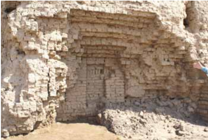
FIGURE 4 The pilasters and exterior facade of the first-phase construction visible within the core of the west wall and partly repaired foundations in 2007. Photo: R. Jaeschke
