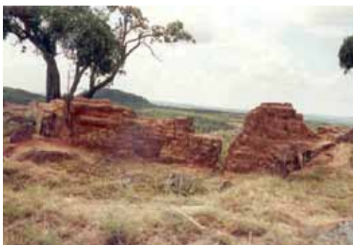
FIGURE 3 Effects of both wind erosion and rain on a daga wall at Nalatale National Monument, Zimbabwe. Photo: Ashton Sinamai
