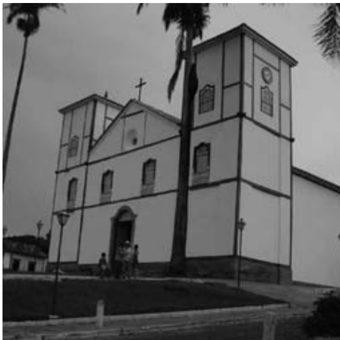
FIGURE 3 Igreja do Rosário (Rosário Church) in Pirenópolis, Brazil, built in the eighteenth century with rammed earth and adobes. Photo: © Honório Nicholls Pereira
