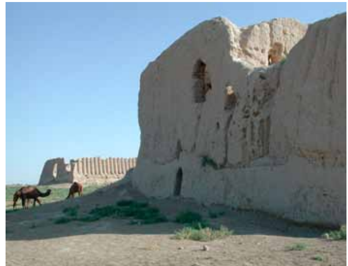
FIGURE 1 The greater and lesser Kyz Kala in Merv, Turkmenistan. Note the repairs at the base of the walls. Photo: Gaetano Palumbo. © World Monuments Fund
