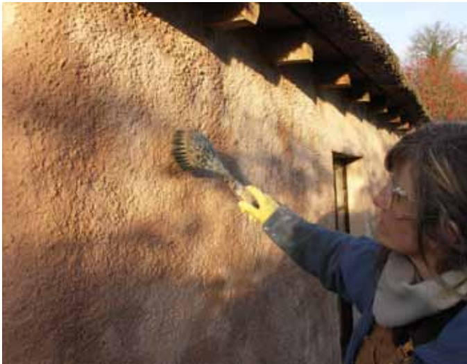
FIGURE 8 Cottown Schoolhouse: application of the final limewash.
