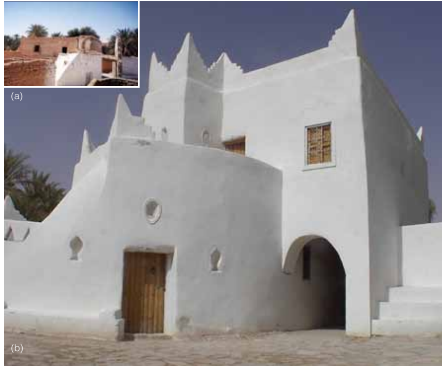
FIGURE 3 Project for the rehabilitation of Ghadames Tylawaan school (a) before and (b) after. Photo: A. Abufayed
