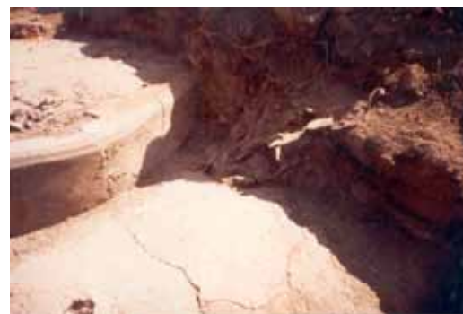
FIGURE 4 When daga structures are exposed the surface cracks almost immediately. These cracks, which were not visible on the structure when it was excavated, appeared after one hour of exposure, Kagumbudzi, Zimbabwe. Photo: Ashton Sinamai
