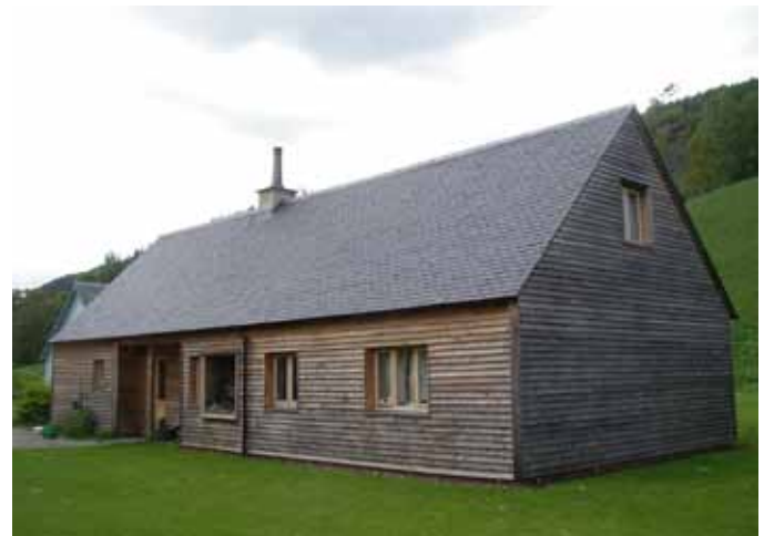
FIGURE 3 Modern timber frame and unfired clay brick building, Dalguise, Scotland. Photo: P. Walker
