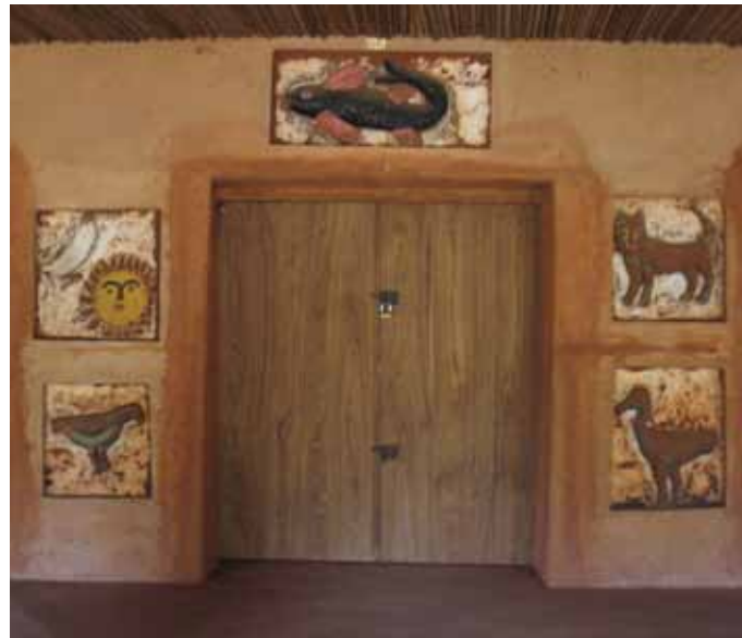
FIGURE 8 Following the Abomey Project, the bas-reliefs from the Ajalala of King Behanzin were conserved by the former site conservator, one of the conservation technicians trained on the Abomey Project, with assistance from local youth. The conservation of these bas-reliefs followed the approach used for the conservation of those from the Ajalala of King Glélé. Photo: Leslie Rainer. © J. Paul Getty Trust, 2006
