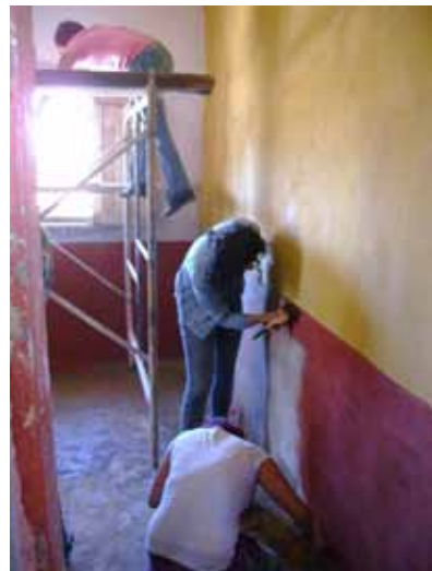
FIGURE 7 Students applying the traditional lime paint in the interiors, El Sauz, Chihuahua, Mexico. Photo: Luis Fernando Guerrero Baca, 2007
