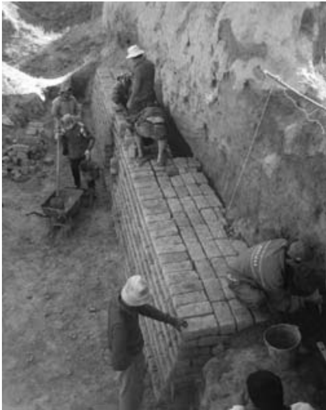
FIGURE 8 Construction of shelter wall against erosion. Spring 2007. Photo: Enrico Fodde
