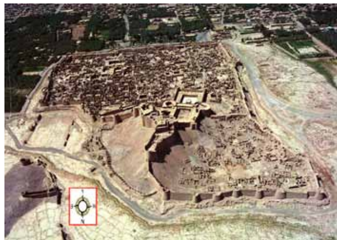
FIGURE 1 The Bam Citadel, aerial image before the earthquake of December 2003.
