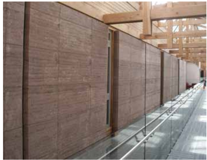
FIGURE 2 Rammed earth wall, Rivergreen Centre, Durham. Photo: P. Walker
