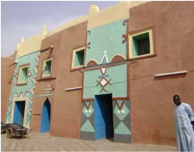
FIGURE 3 Courtyard within the Daura palace complex, January 2008. The paints applied on the wall are of industrial origin. Photo: Ishanlosen Odiaua
