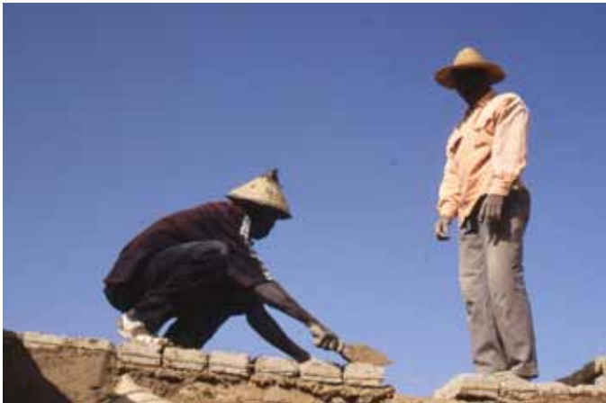
FIGURE 4 Masons constructing a brick wall. Photo: T. H. J. Marchand
