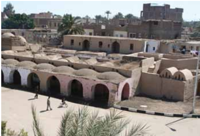
FIGURE 4 A view of part of New Gournna from the minaret of the mosque in 2008. Mud buildings that were built by Hassan Fathy are in a bad state of conservation. Many buildings were replaced by new reinforced concrete blocks. Photo: Hossam Mahdy
