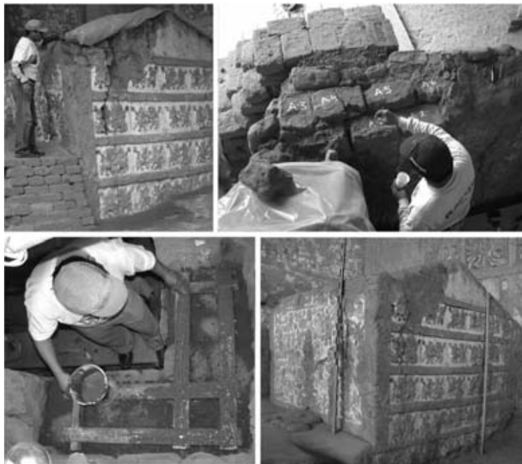
FIGURE 5 Structural reinforcement in walls affected by seismic activity in archaeological times.
