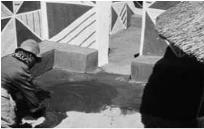
FIGURE 3 Example of a corridor ( umkgothana ) between the front and rear courtyards. The woman who kneels in the frontal section is applying cow dung to the floor. Photo: C. J. van Vuuren
