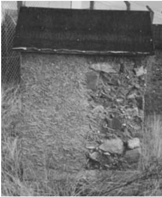
FIGURE 2 ESRP earth-rendered wall: showing only washing away of surface fines after seven years of exposure.
