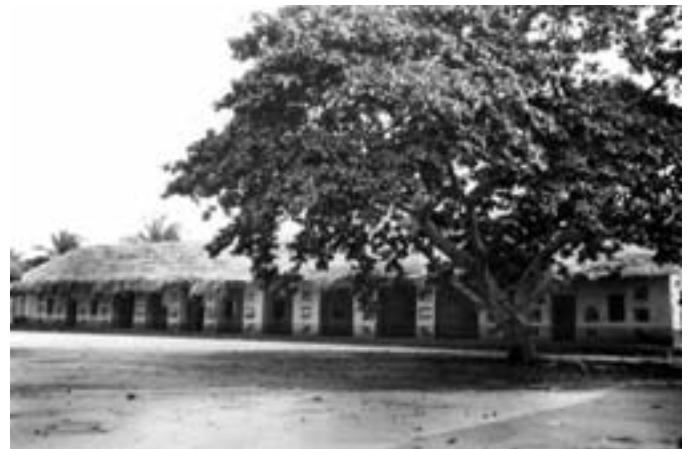
FIGURE 1 Ajalala of King Glélé before the original building was razed and reconstructed. The bas-reliefs on its facade tell the rich history of the Fon people of the Dahomey Kingdom through representations of mythical and symbolic animals, weaponry, and battle scenes. Photo: Eva or Herbert V. Meyerowitz. Courtesy of the Museum of African Art, Smithsonian Institution, Eva Meyerowitz Collection, Eliot Elisofon Photographic Archives, 1937
