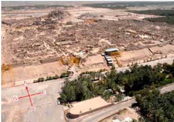
FIGURE 2 The Bam Citadel, aerial image, July 2007. Conservation measures after the earthquake.
