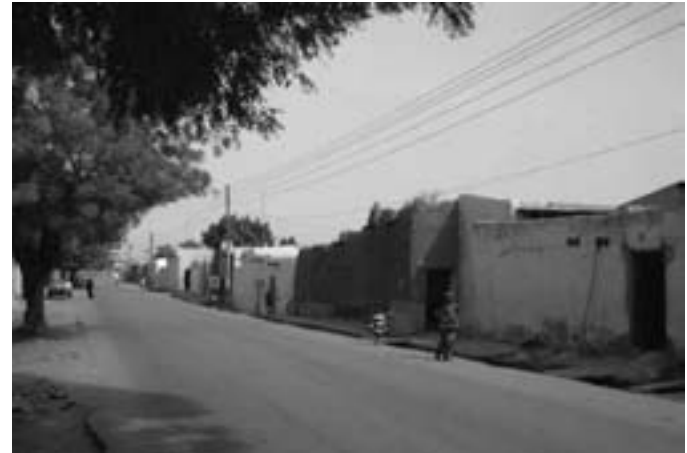
FIGURE 2 Street scene in Daura, January 2008. All the buildings on this street are of earth, plastered over with cement mortar. Photo: Ishanlosen Odiua
