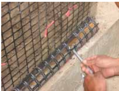
FIGURE 1 Piece of geo-grid. Photo: Daniel Torrealva
