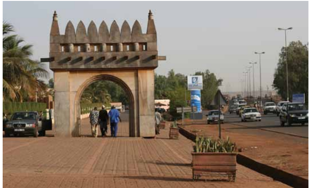
FIGURE 6 Reconstruction of a Djenné-style monumental arch in plywood sheeting on a main road in Bamako. Photo: T. H. J. Marchand
