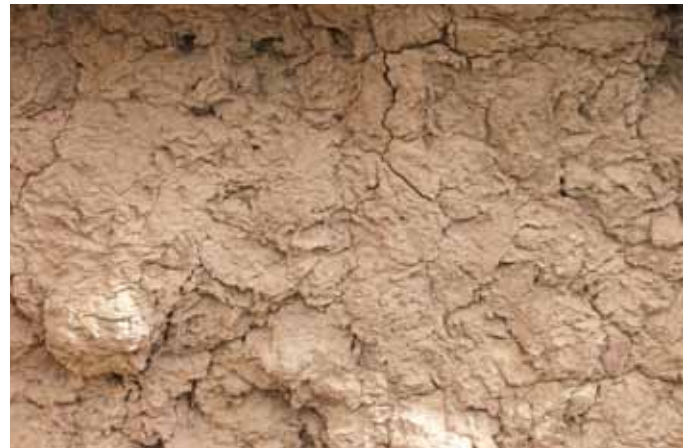
FIGURE 7 Cottown Schoolhouse: the surface was highly degraded, silty, very friable, and lacking in stones or straw.
