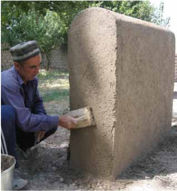
FIGURE 6 Test wall construction. Fall 2006. Photo: Enrico Fodde
