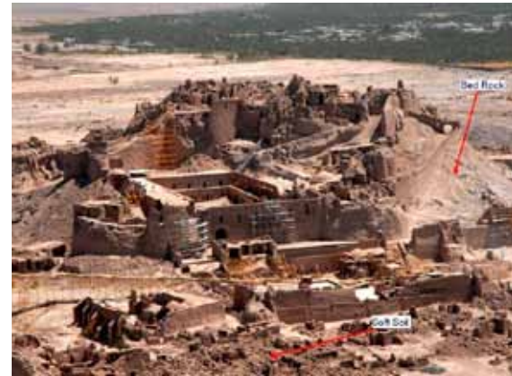
FIGURE 3 Differing extent of destruction in various parts of the Citadel and diverse dynamic behaviors in the bedrock and structures built on soft soil (Caravansarai, Stable, and Payambar mosque).
