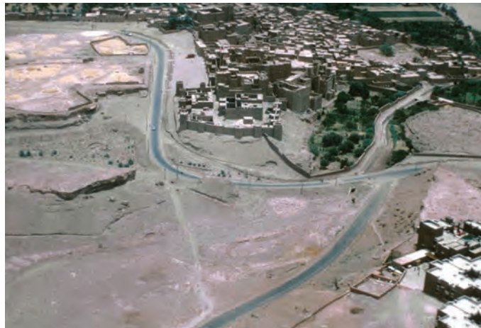
Title: Taourirt, aerial view, 1967-70 est. File name: EAI.MOR.Taourirt.KsarAndKasbah.HistoricImages.CERKAS.IMG_1071.Aerial.jpg Keywords: Taourirt archival image, 1967-70 est., aerial view Copyright: non_JPGT Folder: ArchImg
