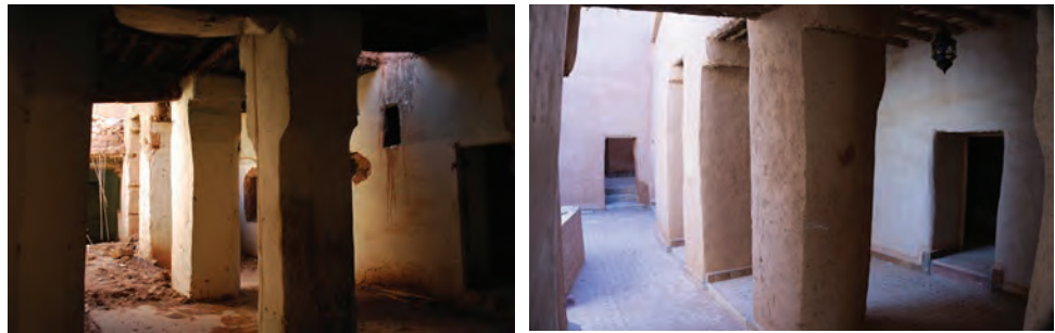
FIGURE K.26A AND K.26B Interior courtyard, Stara East before (left) and after (right) implementation.
