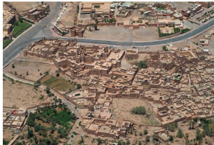
Title: Taourirt, aerial view, 2004 (b) Filename: EAI.MOR.Taourirt.KsarAndKasbah.HistoricImages.CERKAS.IMG_1070.Taourirt.2004.AerialViewB.jpg Keywords: Taourirt archival image, 2004, aerial view Copyright: non_JPGT Folder: ArchImg
