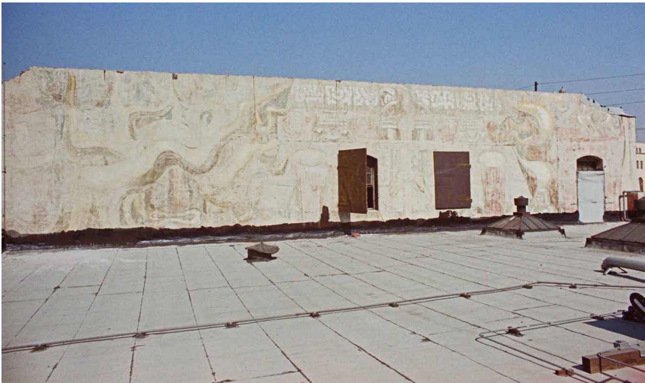
Figure 1 The América Tropical mural in 1971, after the earthquake of February 9, 1971. Earthquake damage can be seen at the upper right and upper left corners. Photo: Jesús Salvador Treviño; mural: © 2012, Artists Rights Society (ARS), New York/Sociedad Mexicana de Autores de las Artes Plásticas (SOMAAP), Mexico City
