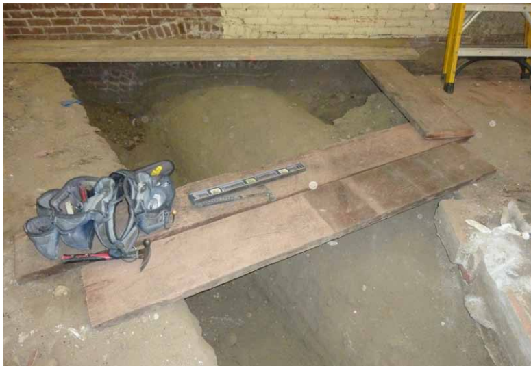
Figure 3 The Zanja Madre exposed during construction. Photo: City of Los Angeles
