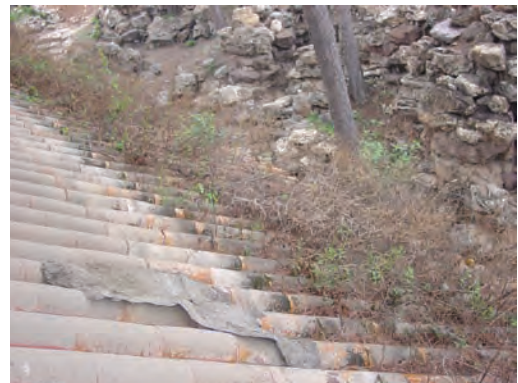
掉在下檐屋顶上的一大片脱落的彩画。 Large pieces of fallen painting on lower eave.
