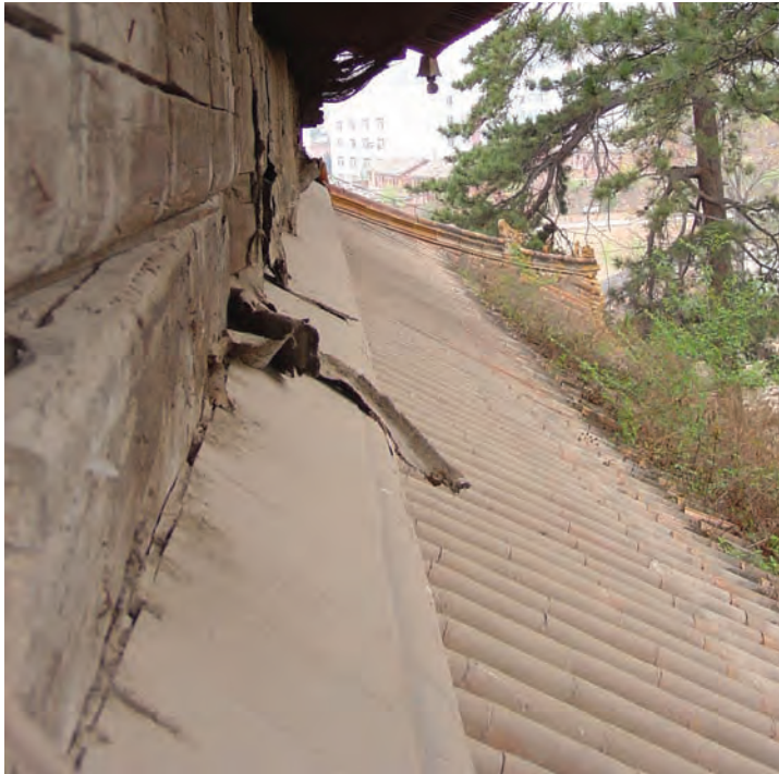
掉在下檐屋顶上的一大片脱落的彩画。 Large pieces of fallen painting on lower eave.
