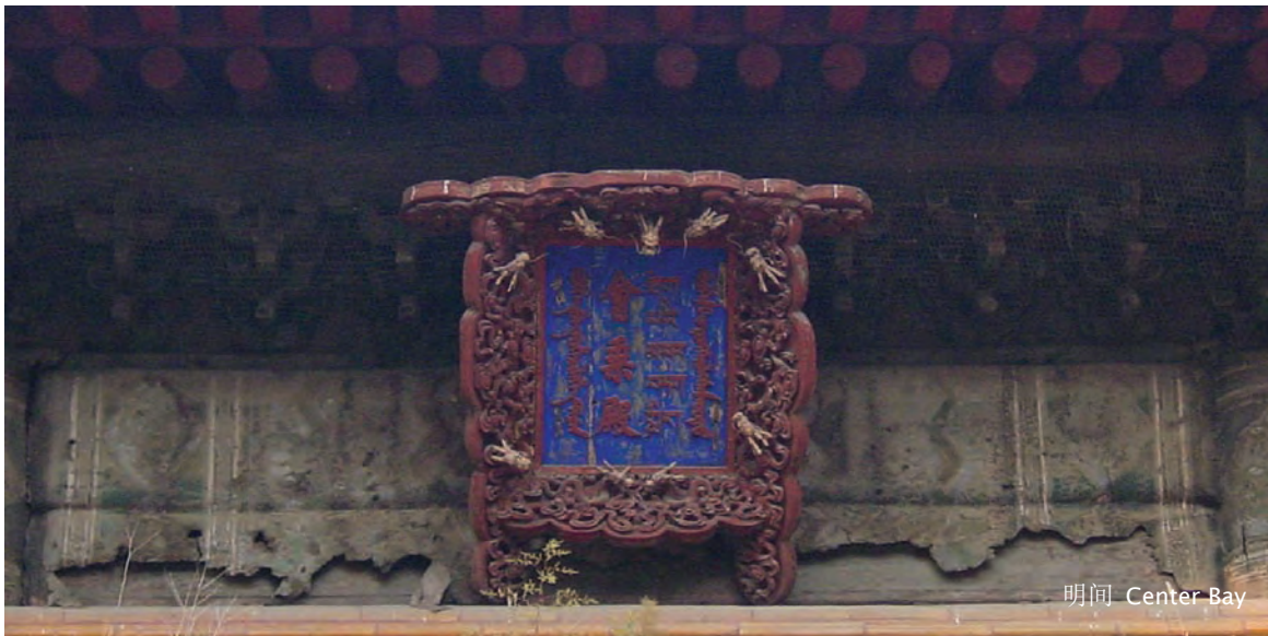
明间：大额枋彩画上有污迹及脏物。小额枋下半部彩画脱落，其余部分有空鼓。几乎所有在斗拱及檩上的彩画都脱落了（照片上看不到）。 Center Bay: greater architrave painting is stained and dirty. The lesser architrave painting is detached and the lower half is lost. Almost all painting is gone on the purlin and brackets (not visible in photograph).
