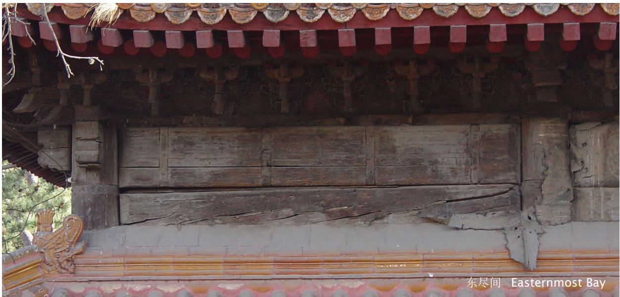
掉在下檐屋顶上的一大片脱落的彩画。 Large pieces of fallen painting on lower eave.
