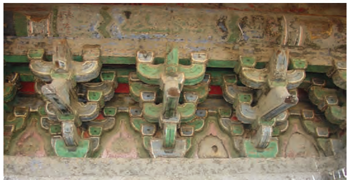
斗拱“蓝绿相间平镏金” Brackets alternate green and blue with a simple gold border decoration
