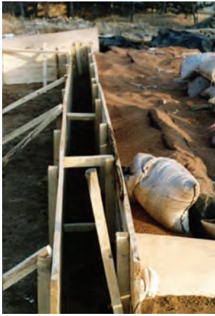
3. 清凉楼，回填用的木结构 Qingliang Building, wooden formwork for reburial
