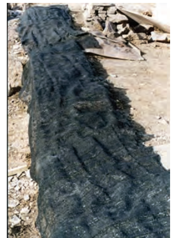
6. 清凉楼，用于回填的分隔层 Qingliang Building, detail of marker layer used in reburial
