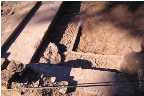
3. 香林室区域，台明石与散水 Xianglin Complex, edge of covered walkway, with drip-line pavement
