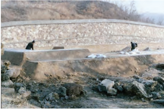
1. 清凉楼，基址回填中 Qingliang Building, reburial in progress
