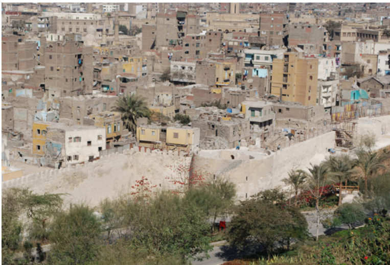
FIGURE 12 The historic center of Cairo, which was conserved with assistance from the Aga Khan Trust for Culture. Photo: Susan Macdonald.
