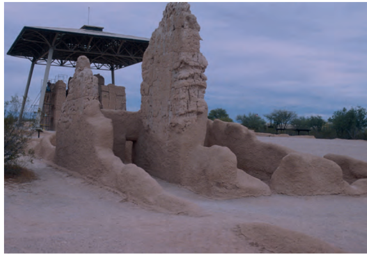
FIGURE 1 Great House, Casa Grande Ruins National Monument, Arizona. Since 1879 both preventive and remedial measures have been taken to preserve this earthen Hohokam site, including the 1902 and 1935 (present) shelters and a continual program of applying amended earthen shelter coats on the exposed low wall ruins. Reproduced by permission of the U.S. National Park Service
