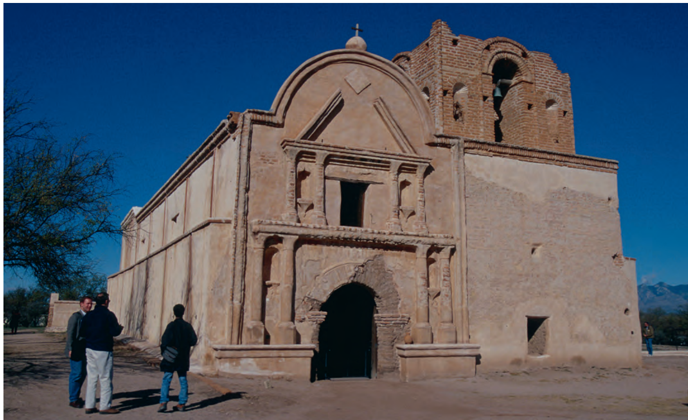
FIGURE 8 Tumacacori, Arizona. Stabilization and early partial reconstruction of the church facade. Photo: Frank Matero
