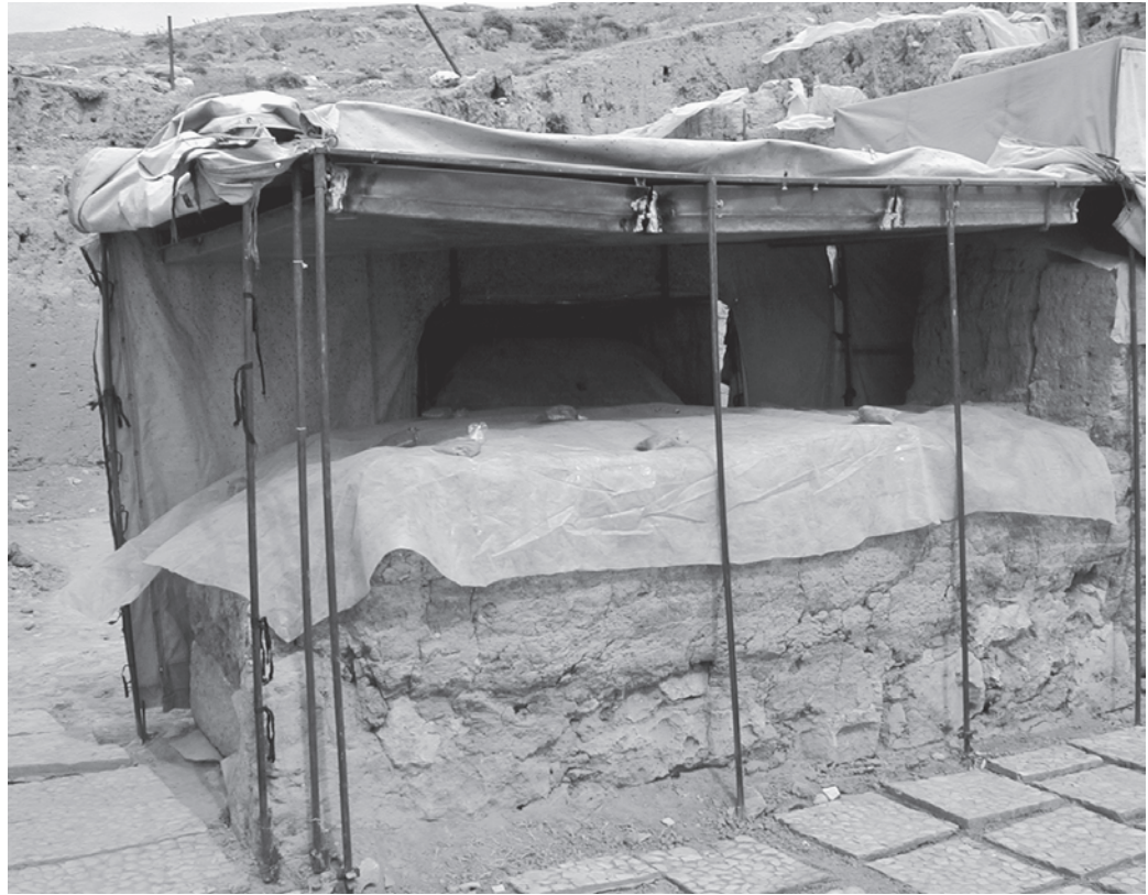
FIGURE 6 Loose plastic cover placed directly on mudbrick, with small sandbags holding it in place, and metal basin at the top to gather water seeping through the tarp (also to hold water in the summer to provide uniform humidity). Photo: G. Buccellati
