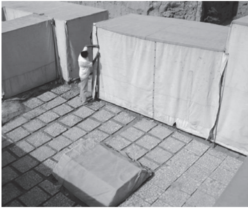
FIGURE 7 Modern pavers in loose and tight arrangement on top of backfill. Photo: G. Buccellati
