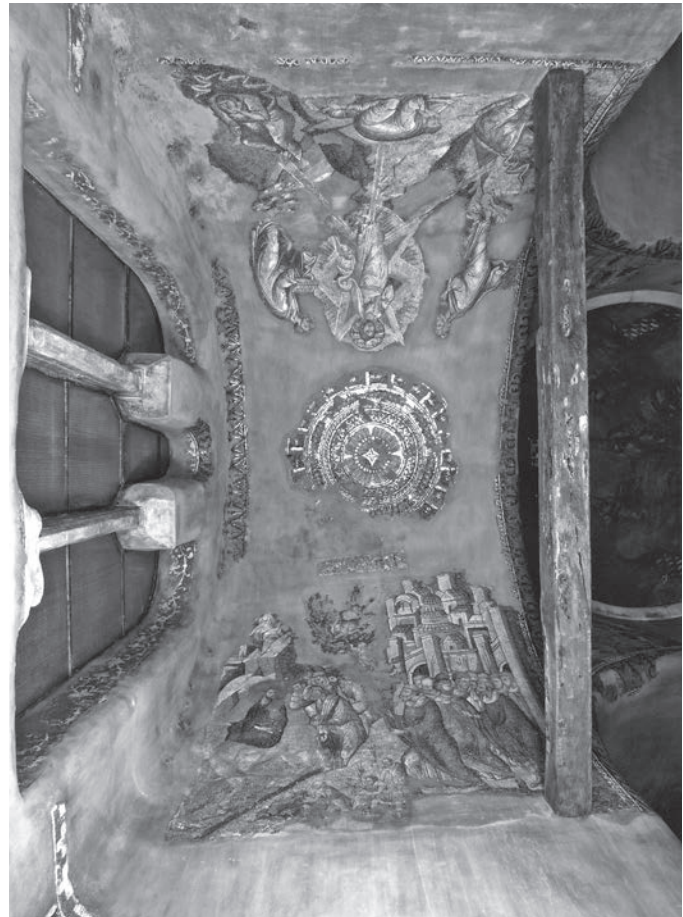
FIGURE 2 The west barrel vault after maintenance treatment. Photo by C. Bakirtzis.
