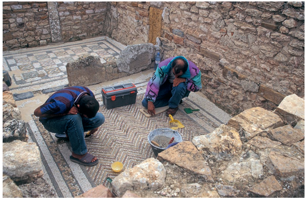
FIGURE 5 Technicians-in-training stabilizing a mosaic pavement at the site of Thuburbo Majus, Tunisia. Photo by Kristin Kelly 2003. © J. Paul Getty Trust.
