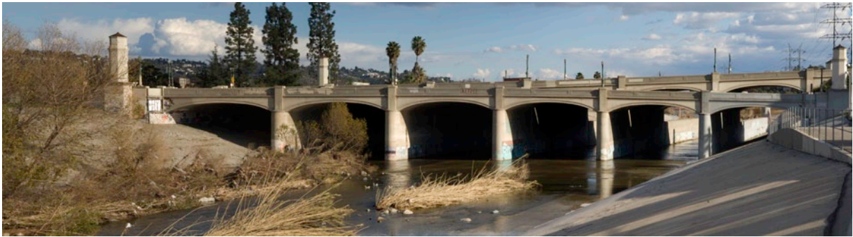
A view of the Glendale-Hyperion Viaduct (HCM #164) from the Los Angeles River. Spanning the river, the 1929 viaduct is constructed of a series of reinforced concrete arches encompassing nearly 1400 feet in length. The survey will identify historic resources such as bridges, street lighting, historic landscapes, and other public works to inform the planning and maintenance of the city's infrastructure. Photo: Emile Askey.
