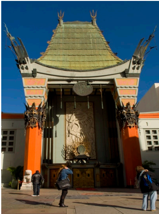
The forecourt of Grauman's Chinese Theatre (HCM #55). An opulent architectural fantasy, Grauman's was the second movie palace in Hollywood when it opened in 1927. It is a contributor to the Hollywood Boulevard Commercial and Entertainment National Register Historic District. The citywide historic context statement would establish the themes, chronological periods, persons, places, and events significant in Los Angeles history. Photo: Emile Askey.
