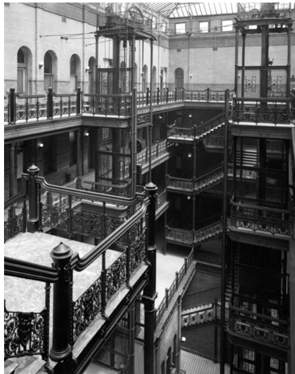
Interior court of the Bradbury Building (HCM #6). Constructed in 1893, the Bradbury is the oldest extant commercial building in downtown Los Angeles. Its significant features include a dramatic interior court, ornamental iron railings, and open-cage elevators, features preserved through the application of the CHBC during a 1990s rehabilitation. Designated as a Los Angeles HCM in 1962, the Bradbury Building is also a National Historic Landmark. Photo: Security Pacific Collection/Los Angeles Public Library.
