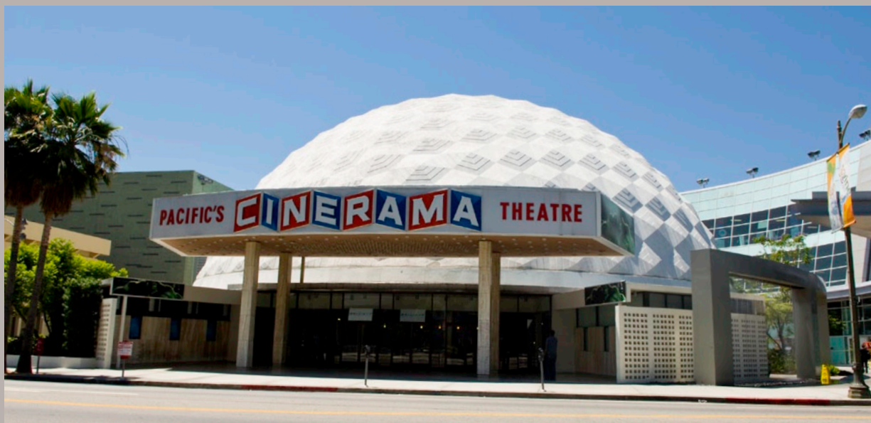
Front entrance of the Cinerama Dome in Hollywood (HCM #659). The design and scale of the new entertainment complex built around this historic, Welton Becket-designed dome was influenced by public dialogue conducted during the environmental review process. When proposed projects require environmental reviews, historic resources must be identified and potential impacts upon them assessed. Photo: Emile Askey.
