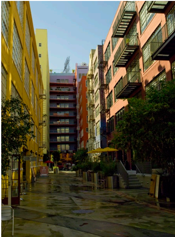
Santee Court (HCM #710 and #711). Under the Mills Act, the developers of Santee Court extensively rehabilitated the former M. J. McConnell Buildings—nine historic garment-manufacturing buildings—into a mixed-use development. Photo: Emile Askey.
