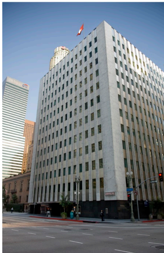
The Standard Hotel (HCM #686) in downtown Los Angeles. Conversion of the 1956 Superior Oil Company Building into the trend-setting Standard Hotel employed both a $7.2 million Federal Rehabilitation Tax Credit and the Los Angeles ARO, reducing development time and costs, taxes, fees, and other development expenses. Property owners can rely on historic resource survey data to shape plans for their property, including the use of incentives. Photo: Emile Askey.
