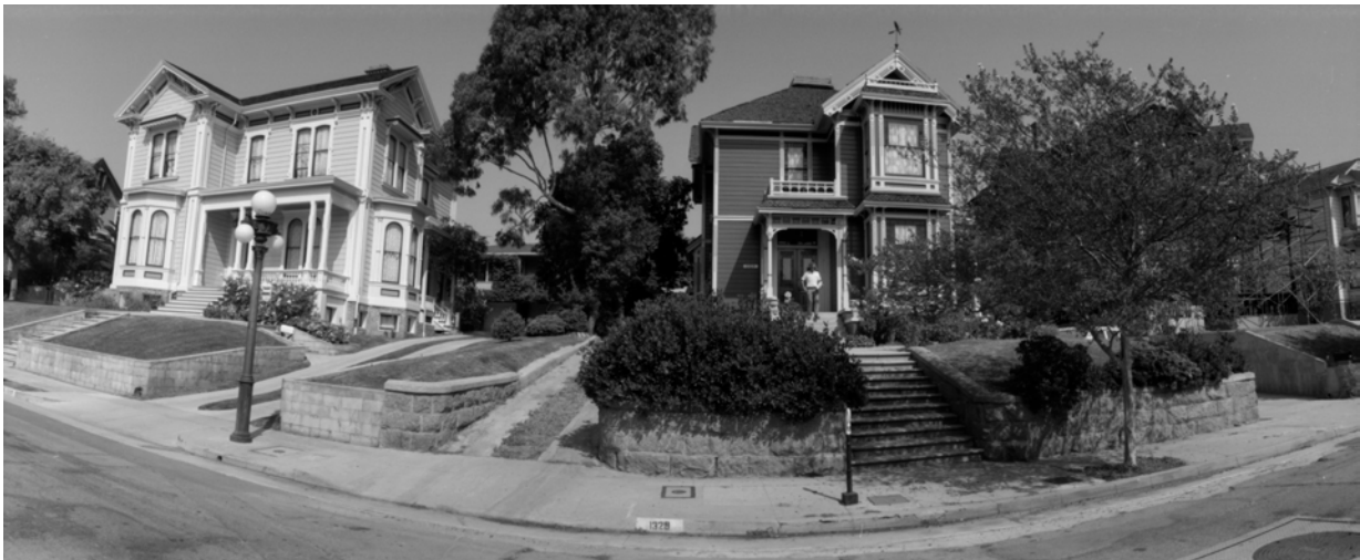
Homes in the Angelino Heights HPOZ. This area was designated as the city's first HPOZ in 1983, initiated by property owners who wanted to preserve and enhance the historic character of their neighborhood, which contains some of the city's best remaining examples of Victorian architectural styles. The HPOZ designation process involves property owners extensively and may serve as a model for survey participation. Owners will be able to contribute to and obtain information from the survey regarding the historic merit of their properties. Photo: John C. Lewis.
