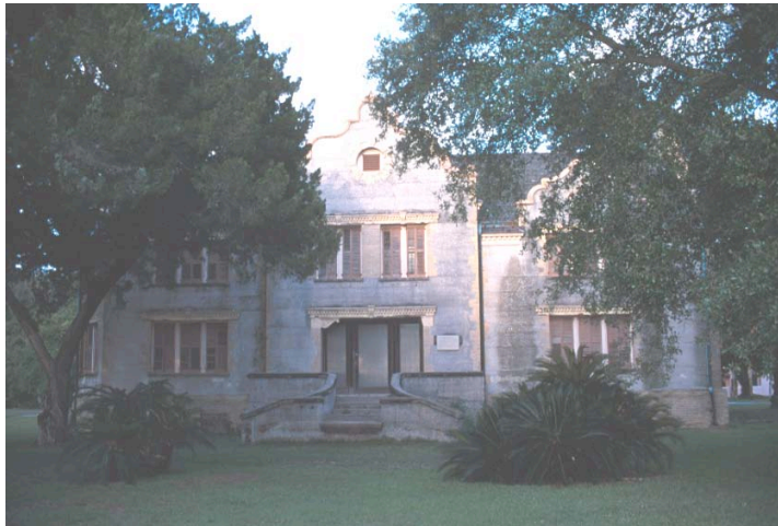
Figure 1 Main (west) façade of Hollybourne Cottage.
