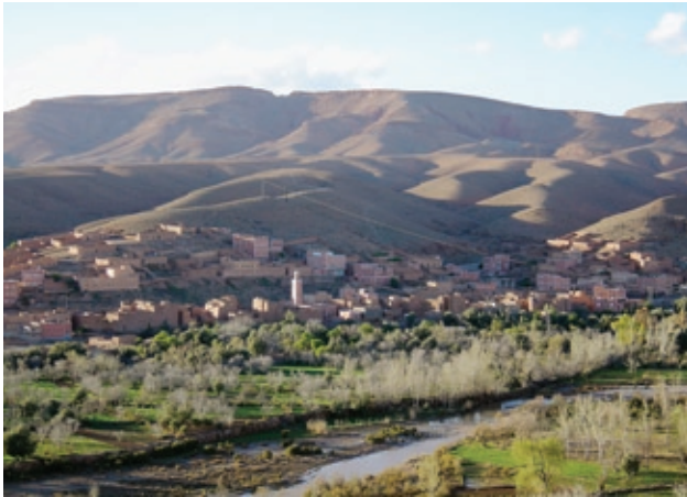
FIGURE 5 New houses sprawling away from an old qsar , Tissergat, province of Ouarzazate.
