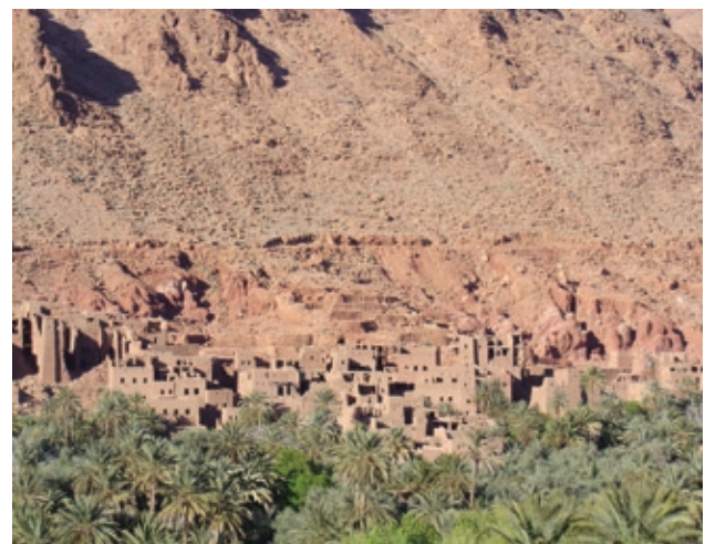
FIGURE 4 An abandoned qsar (a walled earthen town settlement), Tineghir, province of Ouarzazate.
