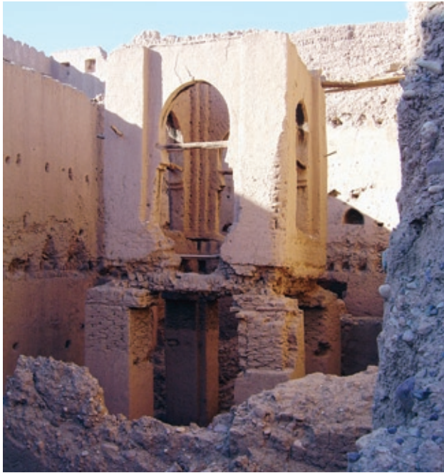
FIGURE 6 Remains of a four-column structure.
