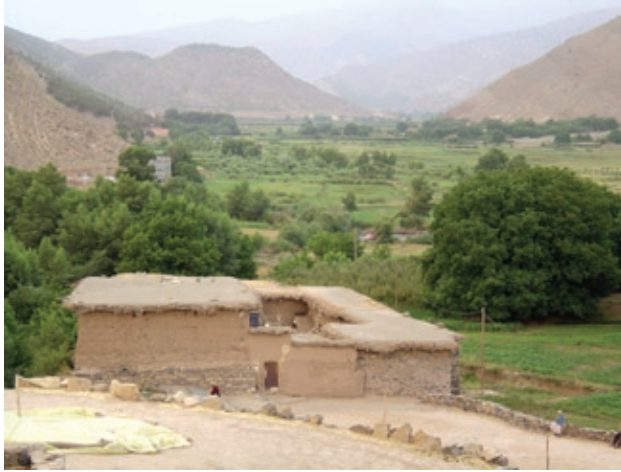
FIGURE 9 New house, Ait Bouguemmaz.
