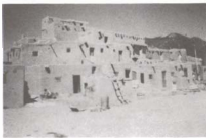
Figure 1. Five-story Taos Pueblo originally built of puddled adobe (made by patting mud into a wall-shape) before the introduction of Spanish adobe forms. Note mud plastering that is carried out each year to maintain the structure.
