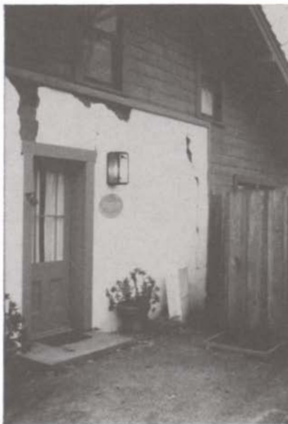
Figure 2. North end wall, Branciforte Adobe, 1990
