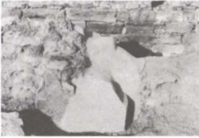
Figure 5. Section/pier of Megaron 1 after mud plaster application.
