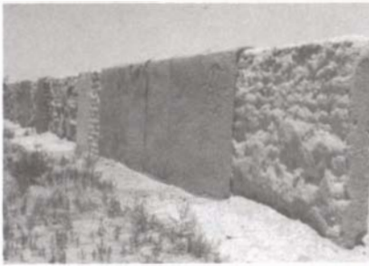
Fig. 7 Amended wall west face. Control panel is on the right.
