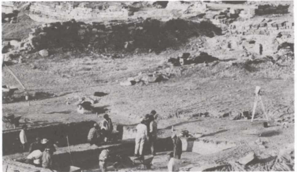
Figure 4. Overall deterioration of Megaron 1.
