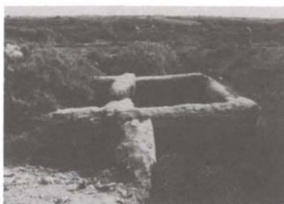
Figure 14. Two rooms at "Via Porticata" which were protected with the soil-cement capping. In this case the capping performed better, probably because people did not walk over it.
