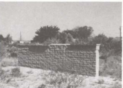
Fig. 5 Wall cap experiment, looking northwest.
