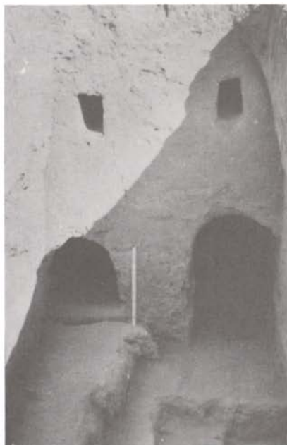
Fig.4. Lobby with two doors and two windows for the stair-case. Early 8th century.
