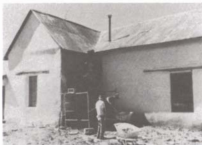
Figure 5 Work in Progress La Capilla de San Antonio Chacon, New Mexico
