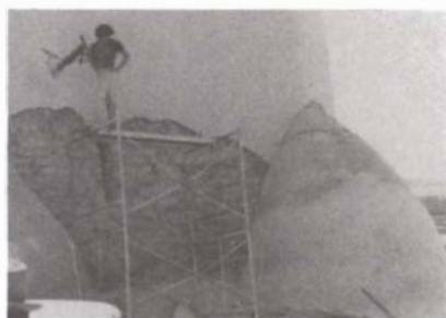
Figure 14 Removing Cement Stucco Before Mud Plaster San Francisco de Assisi Ranchos de Taos, New Mexico
