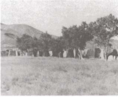
Preservation landscaping. Grass was planted on the parade ground to reduce the amount of wind carried abrasives. The trees replicate the historic landscape, 1985. New Mexico State Monuments.
