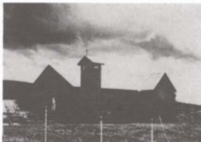
Figure 9 Cement Stucco Removal La Capilla de San Antonio Chacon, New Mexico
