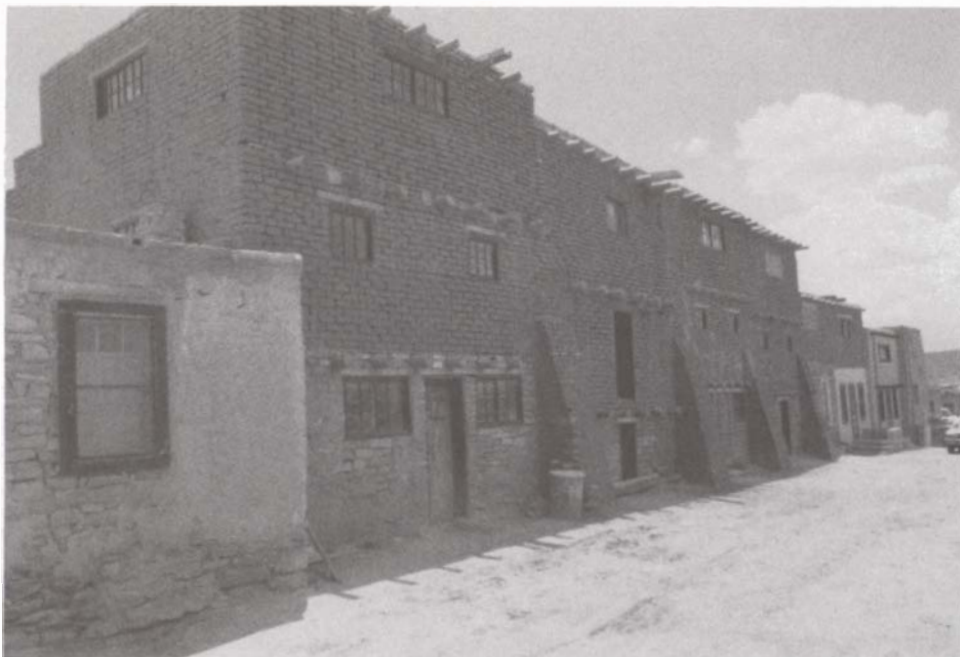
Architectural elements without historical background; buttresses and side by side windows.
