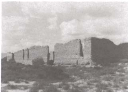
Adobe wall before stabilization, 1974. New Mexico State Monuments.
