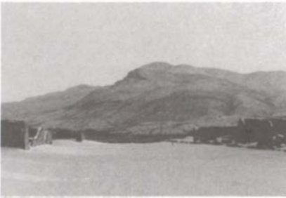
Drainage contours to prevent accumulation of water next to walls. The grade is established to the center of this roadway. After snow, 1974. New Mexico State Monuments.
