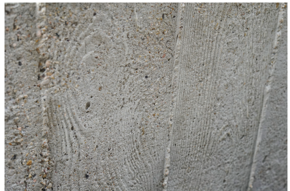
FIGURES 4A–E Examples of concrete finishes: (a) tile cladding on concrete, Sydney Opera House, Jørn Utzon, Sydney, Australia, 1973. Photo: Greg O’Beirne, 2006, licensed under CC BY-SA 3.0 Unported; (b) bush-hammered concrete, Barbican Centre, Chamberlin, Powell & Bon, London, UK, 1976. Photo: Ana Paula Arato Gonçalves, 2019, © J. Paul Getty Trust; (c) ribbed concrete with exposed aggregate. Photo: Ana Paula Arato Gonçalves, 2019, © J. Paul Getty Trust; (d) board-marked concrete. Photo: Ana Paula Arato Gonçalves, 2019, © J. Paul Getty Trust; and (e) concrete mimicking stone, Palais d’Iéna, Auguste Perret, Paris, France, 1937–46. Photo: Ana Paula Arato Gonçalves, 2018, © J. Paul Getty Trust.
