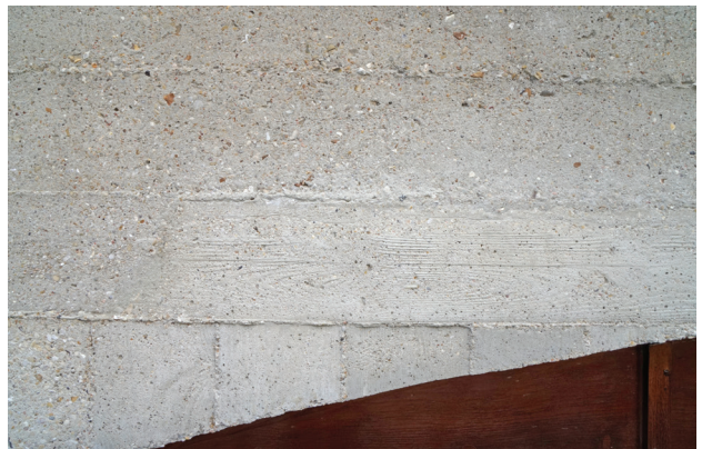
FIGURES 2A, 2B Achieving durable patch repairs that are compatible with the preservation of aesthetic significance of original concrete is a typical challenge in conserving concrete. (a) Example of poor aesthetic match. Photo: Ana Paula Arato Gonçalves, 2019, © J. Paul Getty Trust; (b) example of good aesthetic match. Photo: Ana Paula Arato Gonçalves, 2019, © J. Paul Getty Trust.
