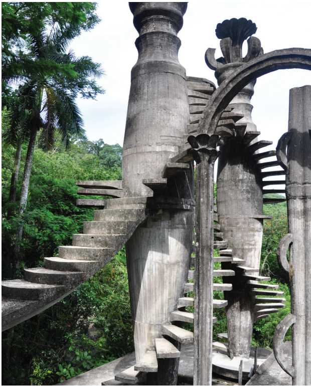
FIGURES 2A, 2B Achieving durable patch repairs that are compatible with the preservation of aesthetic significance of original concrete is a typical challenge in conserving concrete. (a) Example of poor aesthetic match. Photo: Ana Paula Arato Gonçalves, 2019, © J. Paul Getty Trust; (b) example of good aesthetic match. Photo: Ana Paula Arato Gonçalves, 2019, © J. Paul Getty Trust.
