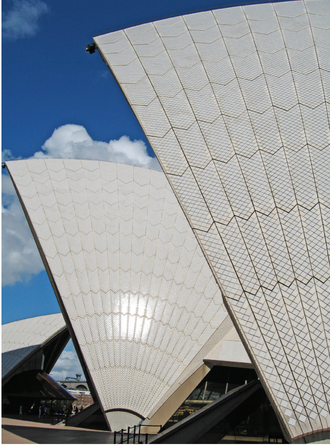
FIGURES 4A–E Examples of concrete finishes: (a) tile cladding on concrete, Sydney Opera House, Jørn Utzon, Sydney, Australia, 1973. Photo: Greg O’Beirne, 2006, licensed under CC BY-SA 3.0 Unported; (b) bush-hammered concrete, Barbican Centre, Chamberlin, Powell & Bon, London, UK, 1976. Photo: Ana Paula Arato Gonçalves, 2019, © J. Paul Getty Trust; (c) ribbed concrete with exposed aggregate. Photo: Ana Paula Arato Gonçalves, 2019, © J. Paul Getty Trust; (d) board-marked concrete. Photo: Ana Paula Arato Gonçalves, 2019, © J. Paul Getty Trust; and (e) concrete mimicking stone, Palais d’Iéna, Auguste Perret, Paris, France, 1937–46. Photo: Ana Paula Arato Gonçalves, 2018, © J. Paul Getty Trust.
