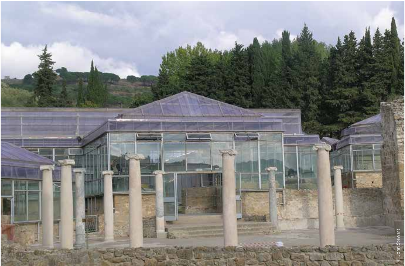
FIGURE 3: The modern ‘glasshouse’ shelter over the Villa Casale at Piazza Armerina, Sicily (Italy) was designed in the 1950s by the architect Franco Minissi, who was influenced by the eminent theoretician Cesare Brandi. It developed iconic status as a modern classic design, and its demolition 50 years later to make way for a new structure with a better internal environment was highly controversial.
