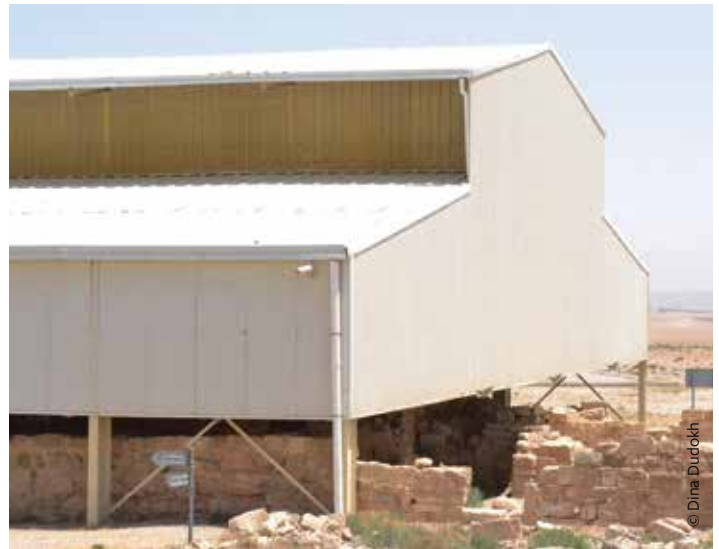
FIGURE 12: Water drainage from the roof surface of the new shelter to ensure that rainwater is collected and channelled away from the complex.
