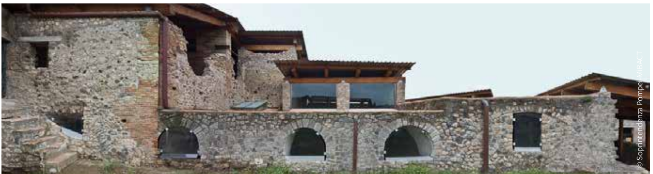
FIGURE 3: An example of a reconstructed compluviate roof in the House of Casca Longus; it has a concrete structure covered by ceramic tiles.
