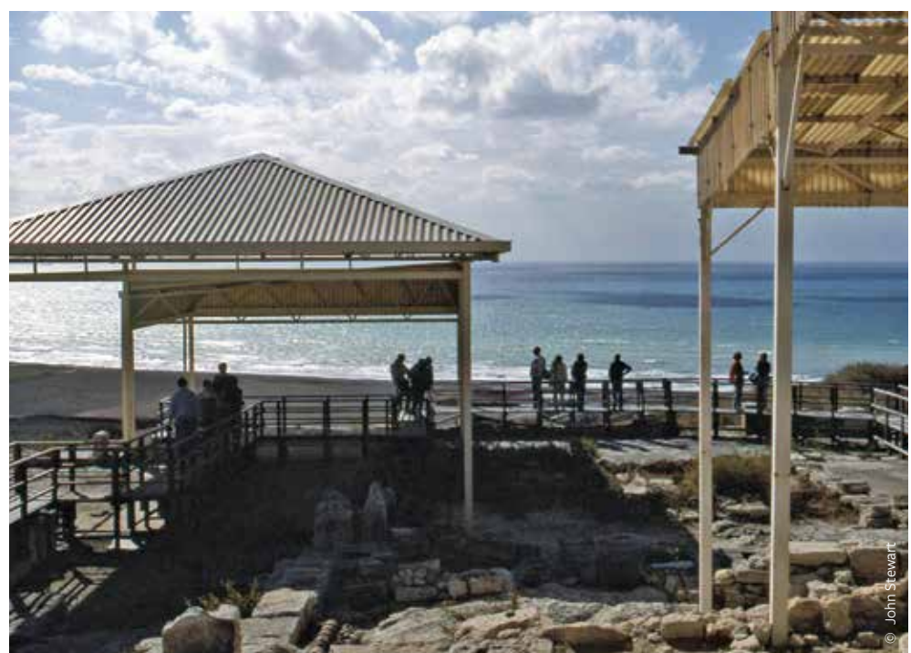
FIGURE 5: The first generation of shelters at Kourion on the coast of Cyprus consisted of open shelters, whose height and span provided no protection for mosaics from raking sunlight or rain.
