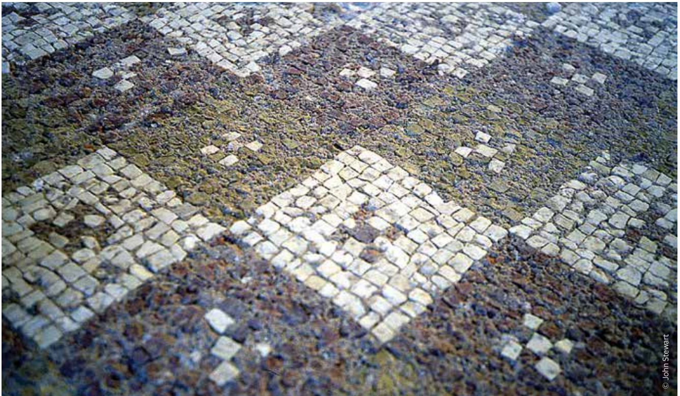
FIGURE 6: Mosaics of the coastal Villa Silin, Libya, in a semi-enclosed room which traps marine aerosols from the sea; they show active deterioration from chloride salts (see the chapter by El-Turki in this publication).
