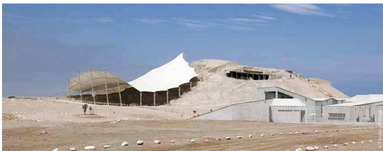
FIGURE 16 (below): The opening of the site to visitors in 2006 prompted the need for several facilities in proximity to the visitor itineraries for Huaca Cao Viejo. In 2009 the Museo Cao was created, where the first more informal visitor facilities had sprung up.
