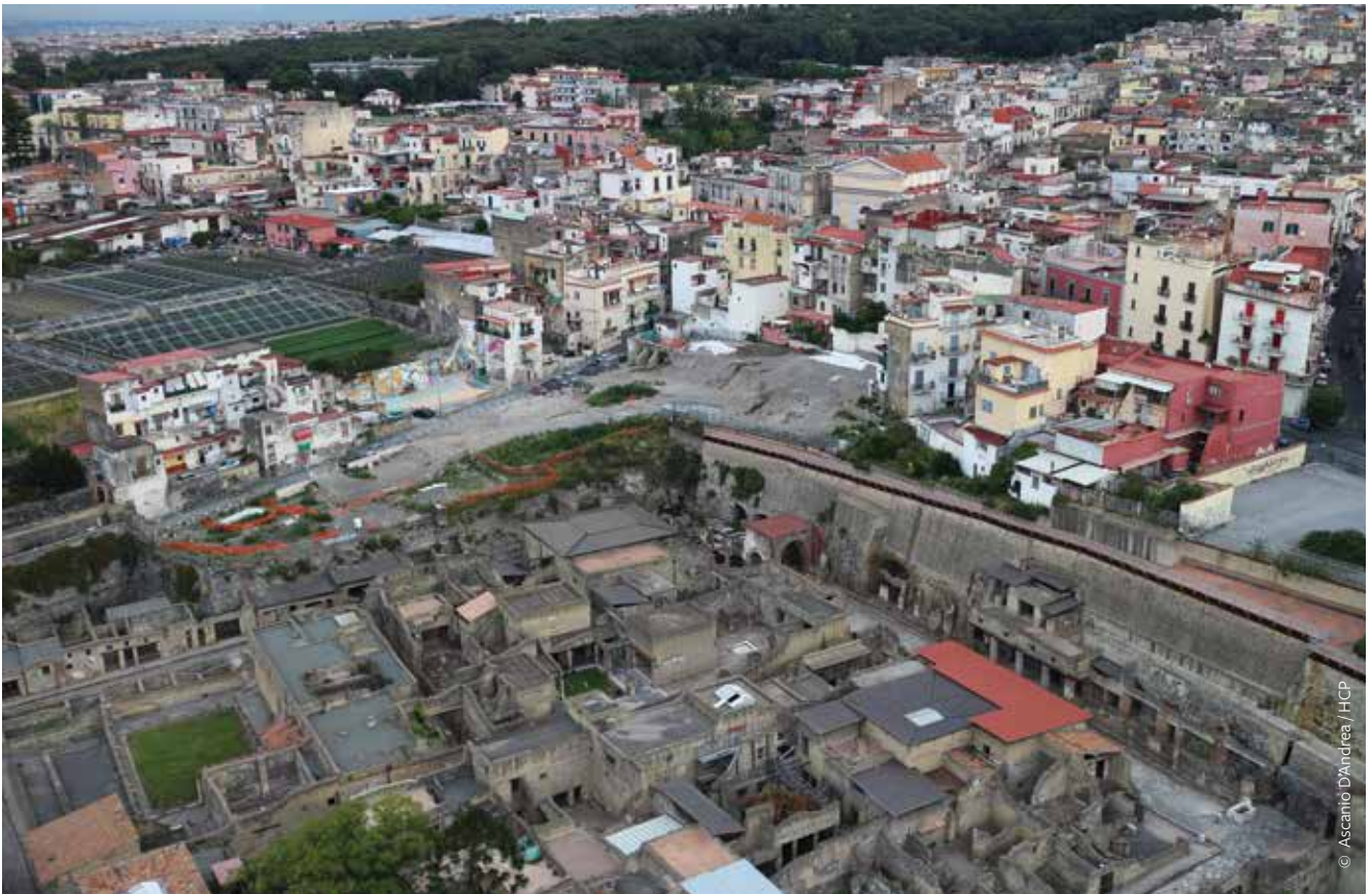
FIGURE 9 (above): The rebuilt roofscape of ancient Herculaneum (Italy) is a mix of reinstated ancient roofs, floor slabs and more abstract shelters where archaeological evidence was lacking. Respecting the spans of the Roman roofs rather than flyover shelters reinforces the legibility of the original urban fabric and reinforces continuity with the modern town above.
