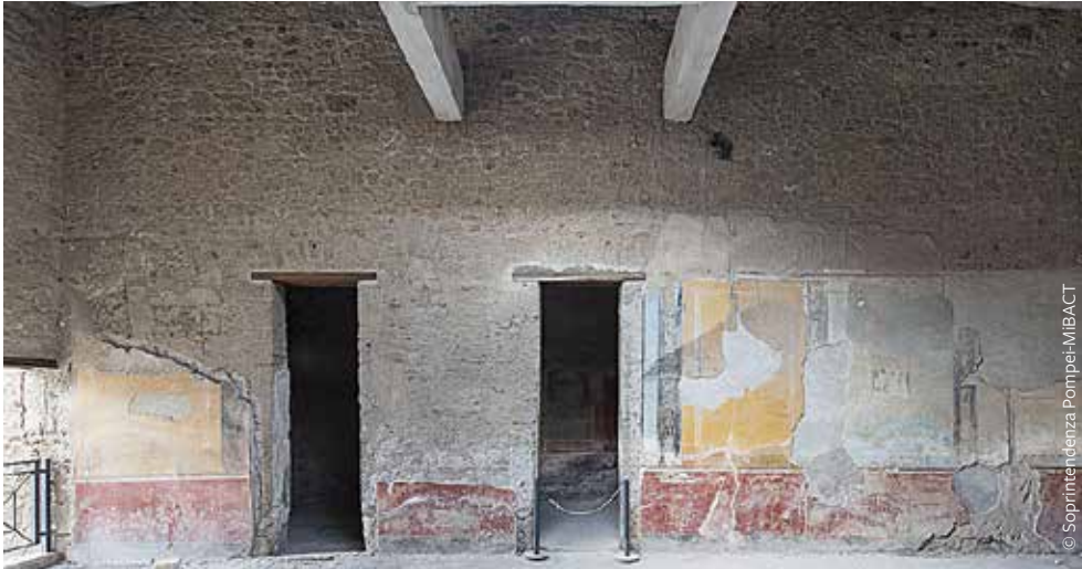
FIGURE 3: An example of a reconstructed compluviate roof in the House of Casca Longus; it has a concrete structure covered by ceramic tiles.
