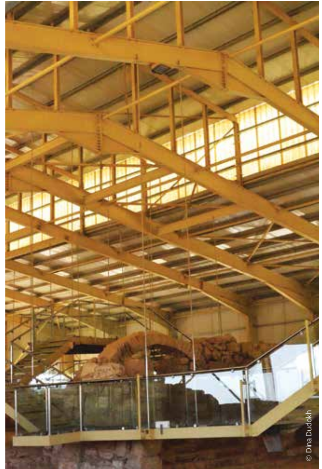
FIGURE 10: The interior of the new shelter at the Saint Stephen's complex, built in 2009. The shape of the roof assists the natural ventilation from the open sides and thus reduces problems of humidity.
