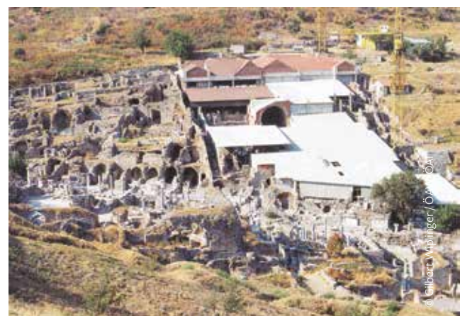
FIGURE 7: The old (1985) shelter over housing units 1 and 2 of Terrace House 2 and temporary shelters over the other units.
