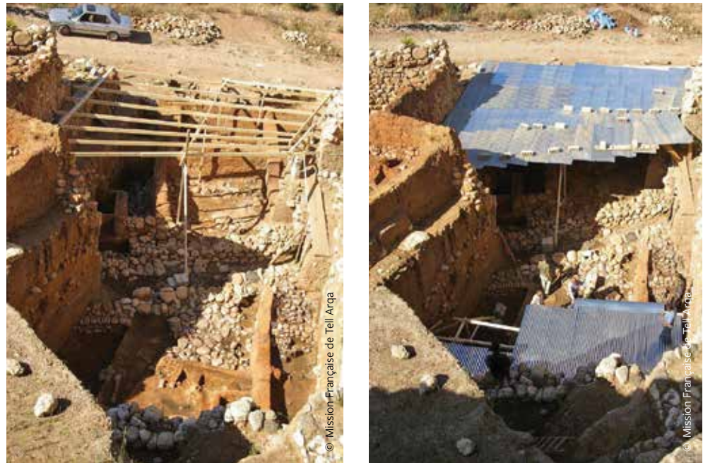
FIGURE 1: Short-term roofing using local materials addresses the limited seasonal nature of climatic phenomena that affect the fragile remains of Tell Arqa (Lebanon) and avoids dependence on more elaborate, hard-to-source building materials.
