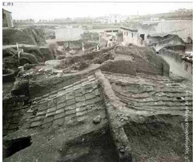
FIGURE 3: Most of the archaeological site of Herculaneum was excavated in the first half of the twentieth century, when teams dug down through the volcanic material to expose the Roman buildings, often finding the original roof structures in situ , although not structurally sound.
