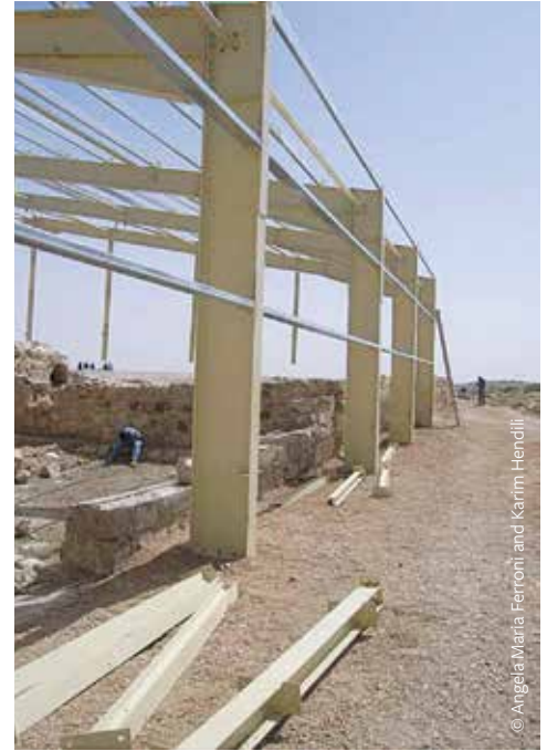
FIGURE 11: Construction of the main new shelter structure, during which protective layers were placed over the mosaic floor.
