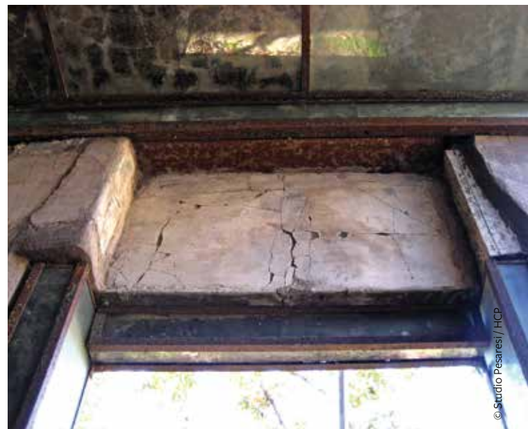
FIGURE 18 (below): Herculaneum: a shelter built in the early 1930s. The shelter's supporting structure also incorporates fragile carbonized wooden panels belonging to the original ceiling. Substituting the entire structure is therefore not an option and a complex intervention of partial substitution/replacement is necessary (see the chapter by Pesaresi and Massari in this publication).
