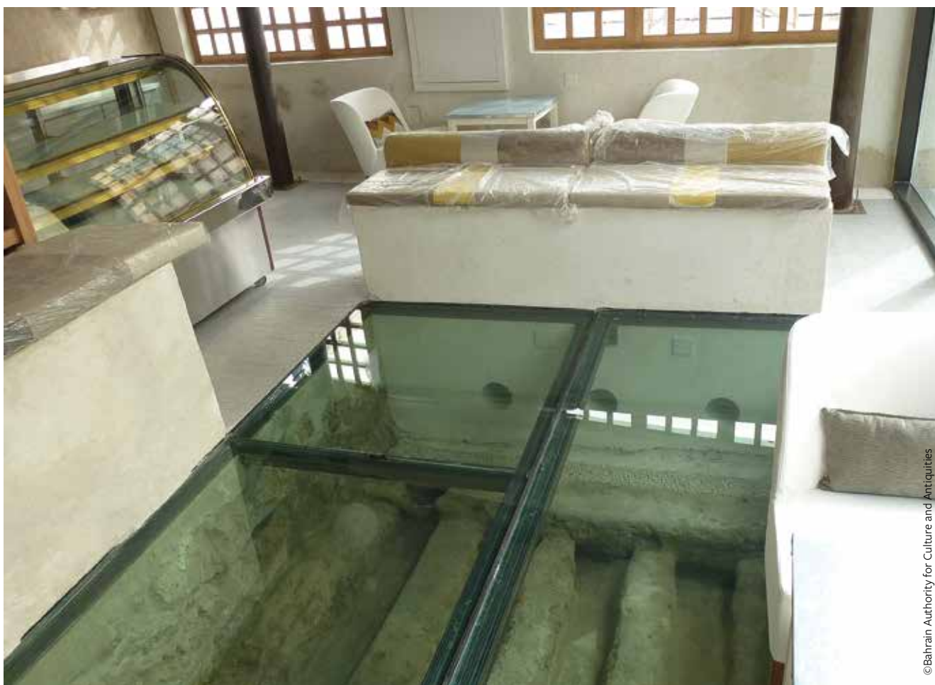
FIGURE 3: The indoor madbasa in 2012 after being revealed and presented in a concealed space roofed with a clear glass. Note the circular holes used for ventilation and the smaller glass pane designed to facilitate access for maintenance.
