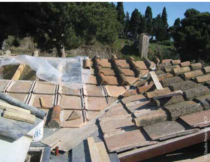
FIGURE 19 (above): An example of corrective maintenance on an ad identicum shelter in Herculaneum: replacement of some of the wooden beams and modification of the system used to channel rainwater away (see the chapter by Pesaresi and Massari in this publication).
