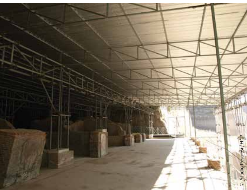
FIGURE 15: A provisional shelter over the Villa of the Papyri, Herculaneum. The supporting structure is built using scaffolding props, the joints of which must be inspected every six months under Italian law. This means the cost of maintenance is extremely high and difficult to carry out, creating significant responsibilities for the site manager.
