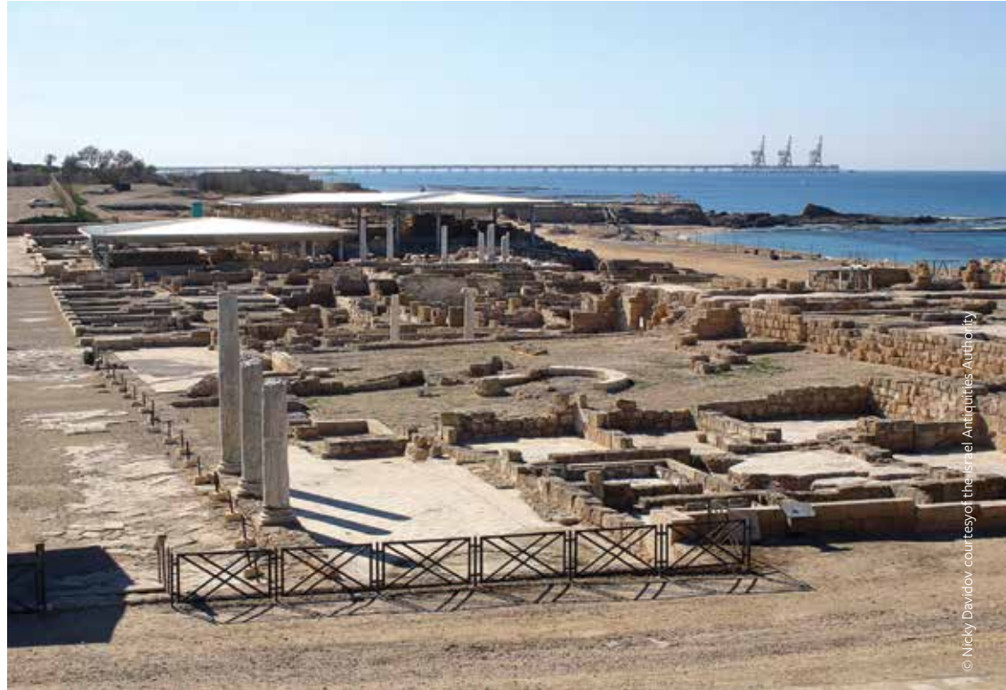
FIGURE 1: In 2001 two large shelters were constructed above the domus and bathhouse in Caesarea. The shelter, situated in a marine environment, protects the mosaics from rain but allows aerosol and dust to accumulate on the mosaic.
