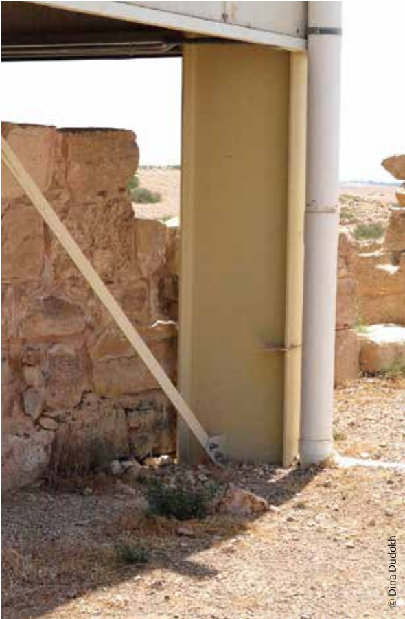
FIGURE 12: Water drainage from the roof surface of the new shelter to ensure that rainwater is collected and channelled away from the complex.
