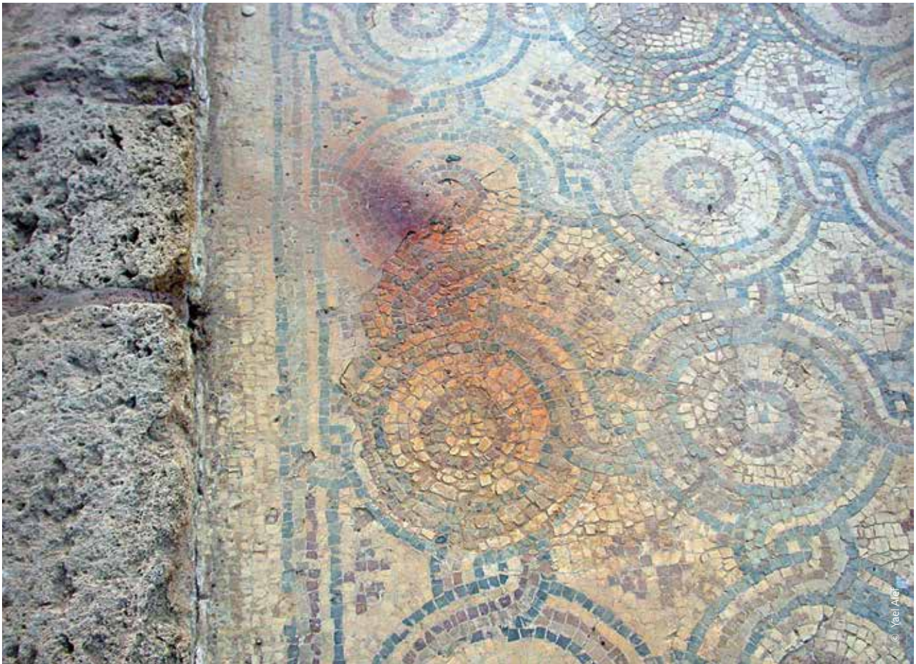
FIGURE 7: Rust stains on the Ibex Mosaic caused by the protective shelter.
