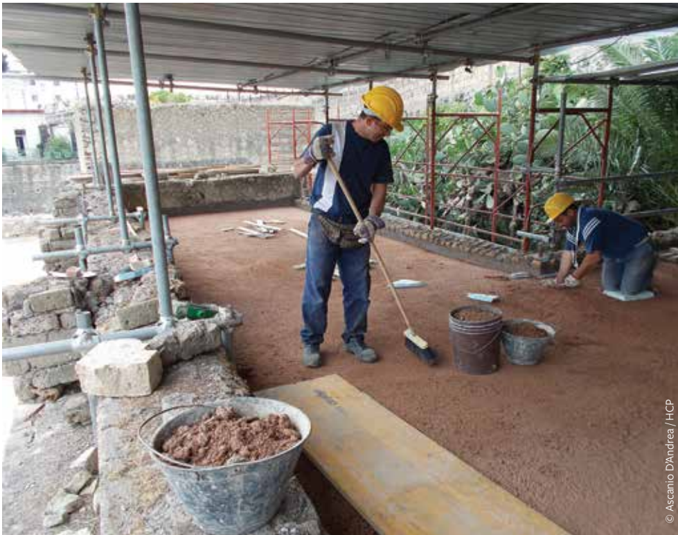
FIGURE 5: When Herculaneum was excavated in the twentieth century some roofs were reconstructed by archaeologists in their original form. These now require periodic maintenance to ensure that they continue their protective function.
