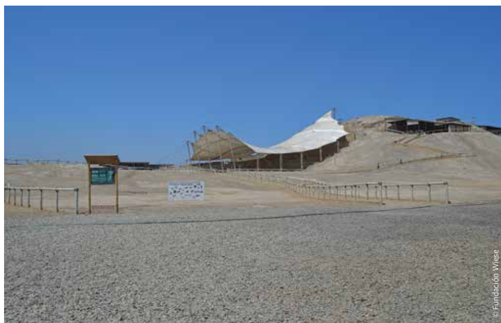
FIGURE 15 (right): Huaca Cao Viejo (Peru) with the tensile structure of 2,500 m 2 , which was erected over the ceremonial square in 2004–05.
