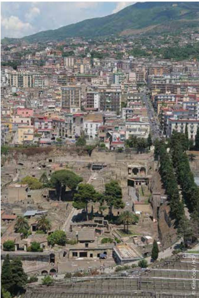
FIGURE 2: The archaeological site lies 20 m below the current ground level and the modern town of Ercolano was built over it from the medieval period onwards. The ability to view the site from above on all sides is a factor that needs to be taken into consideration when designing protective shelters.
