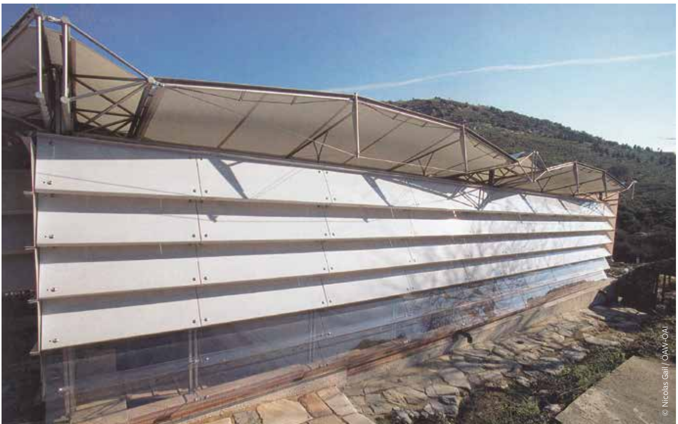
FIGURE 9: Southern view of the shelter where non-transparent panels were used to avoid too much sunlight.
