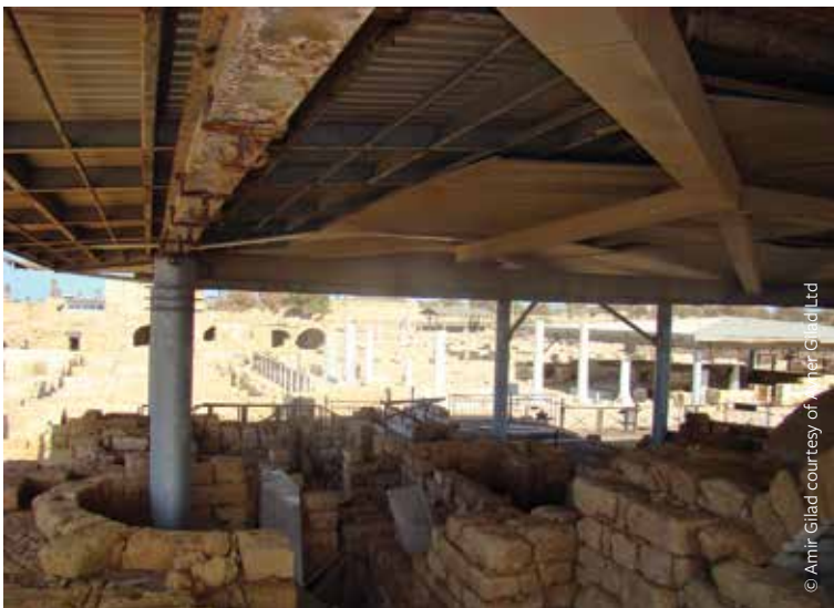
FIGURE 1: In 2001 two large shelters were constructed above the domus and bathhouse in Caesarea. The shelter, situated in a marine environment, protects the mosaics from rain but allows aerosol and dust to accumulate on the mosaic.
