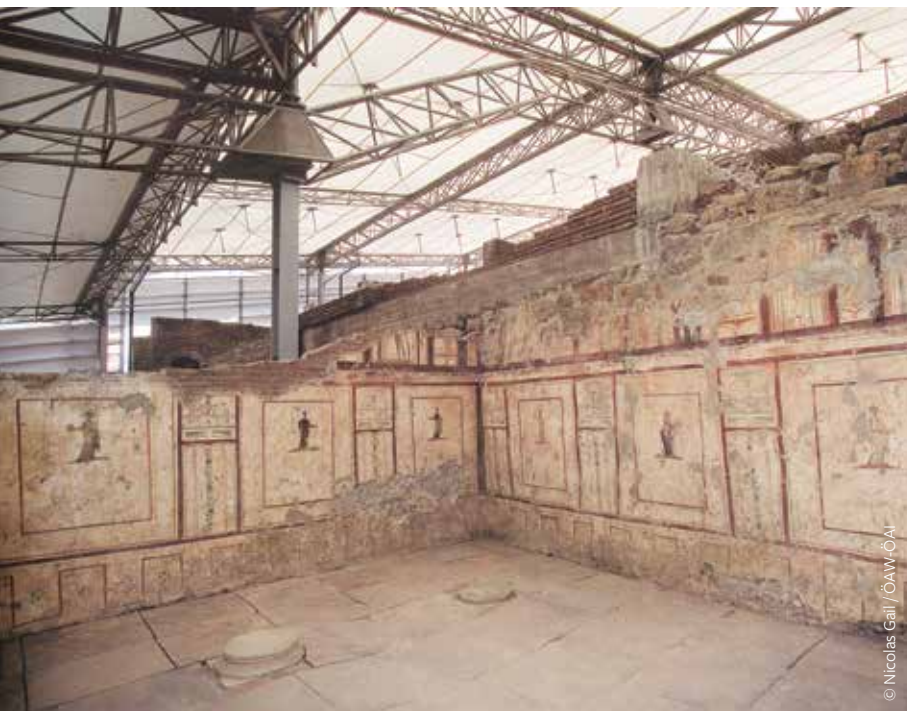
FIGURE 6: Interior view of the shelter over Terrace House 2, from within housing unit 3, room 12.
