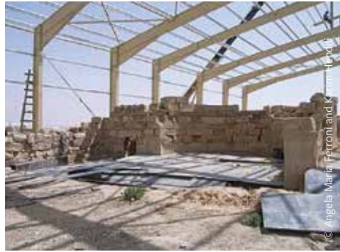
FIGURE 11: Construction of the main new shelter structure, during which protective layers were placed over the mosaic floor.
