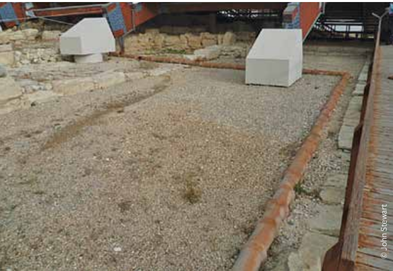
FIGURE 4: The enormous roof over the Annex of Eustolios at Kourion, Cyprus, covers a span of some 35 m, but was designed without drainage. Improvised surface drainage was eventually created with ceramic pipes.
