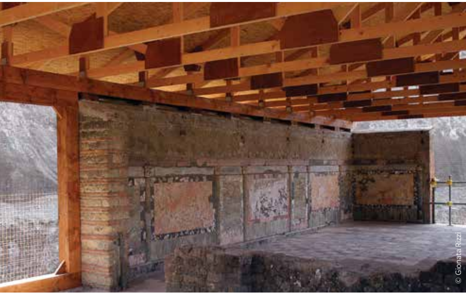
FIGURE 4: New shelter design (above) and construction (left) for the House of the Telephus Relief at Herculaneum (Italy).
