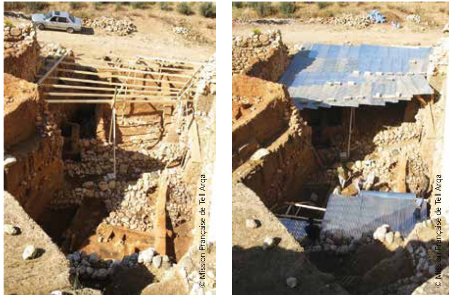
FIGURE 5: The current protective shelters are built on-site each winter using corrugated iron on a timber frame.
