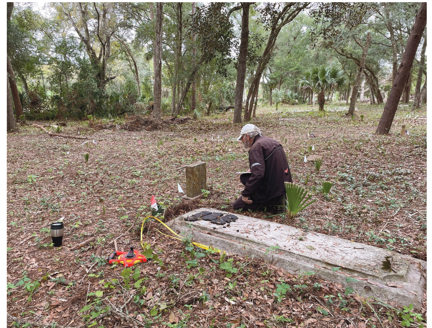
Floodwater can cause the ground to sink, making grave slabs such as these appear to rise or separate from the ground. Oakland Cemetery in Winter Garden, FL. Date taken: 9/29/2020. Photo by FPAN staff member Emma Dietrich.
